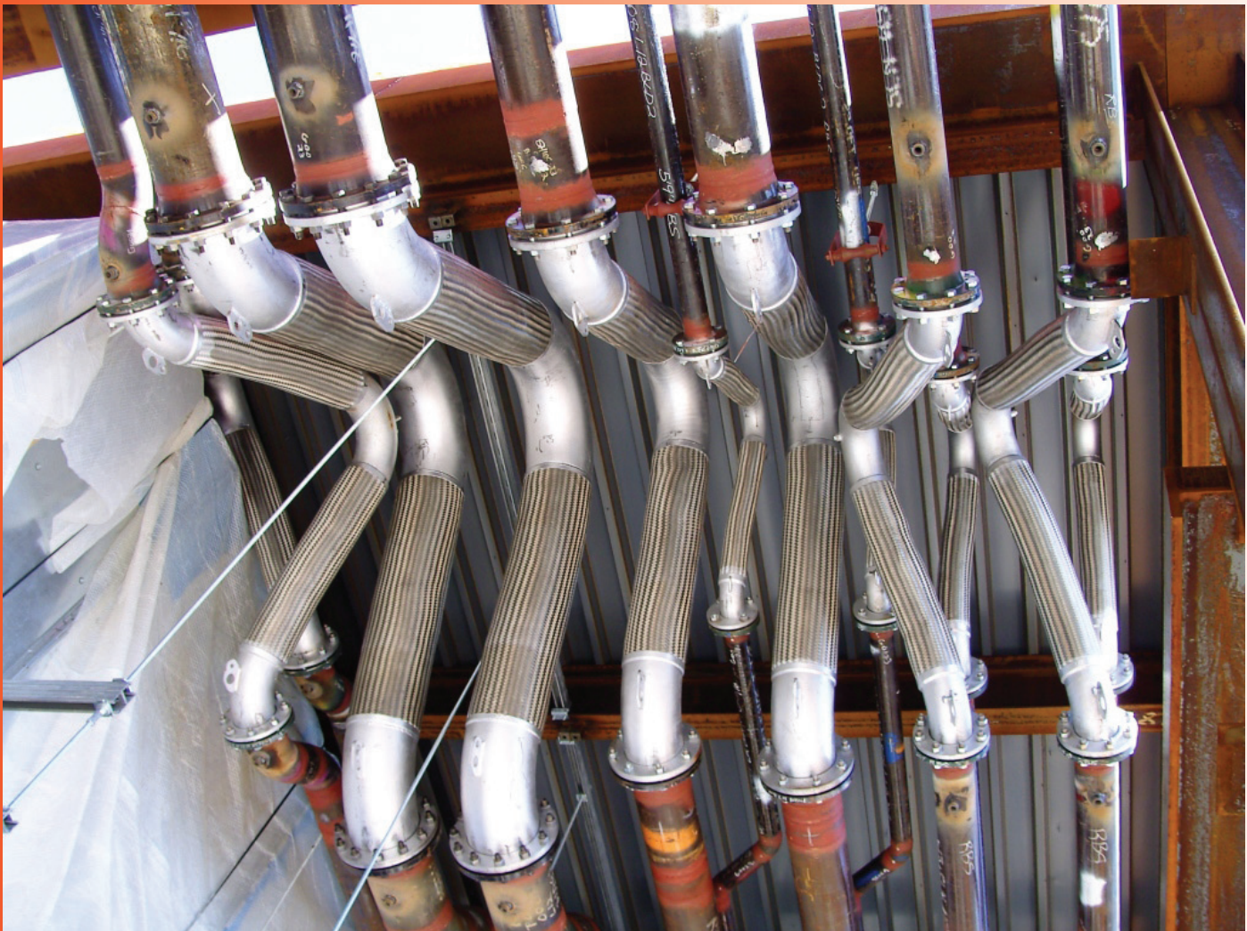
VERTICAL VFL INSTALLATION (Apex Near Ceiling)
